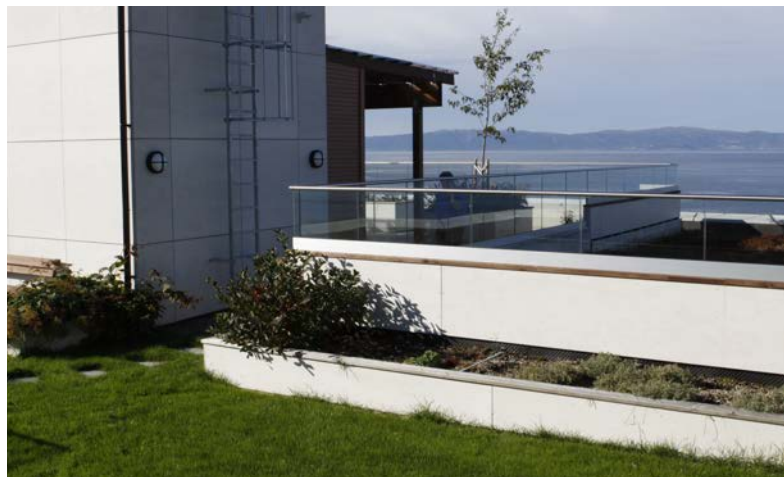
The building of the Malvik facility meets nearly Zero Energy Standards
