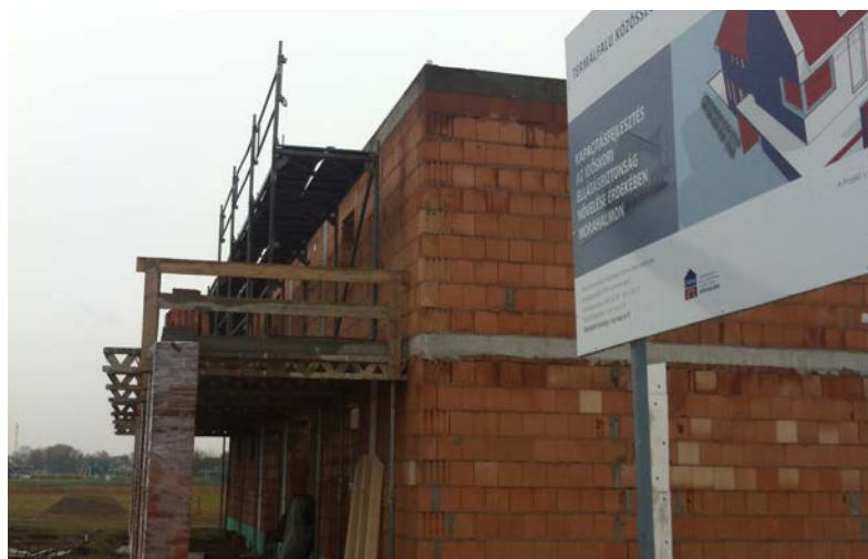
The building of the community house progresses per the original plans
