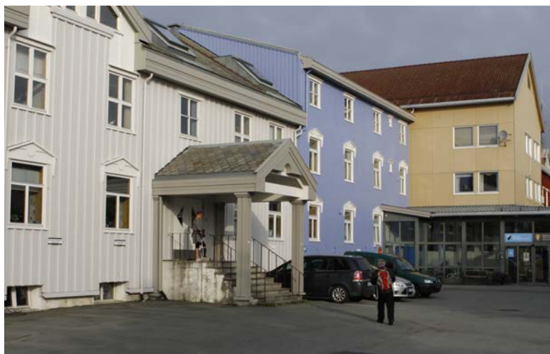
The Fosen facility was built in the 1970s, yet it perfectly serves its many functions
